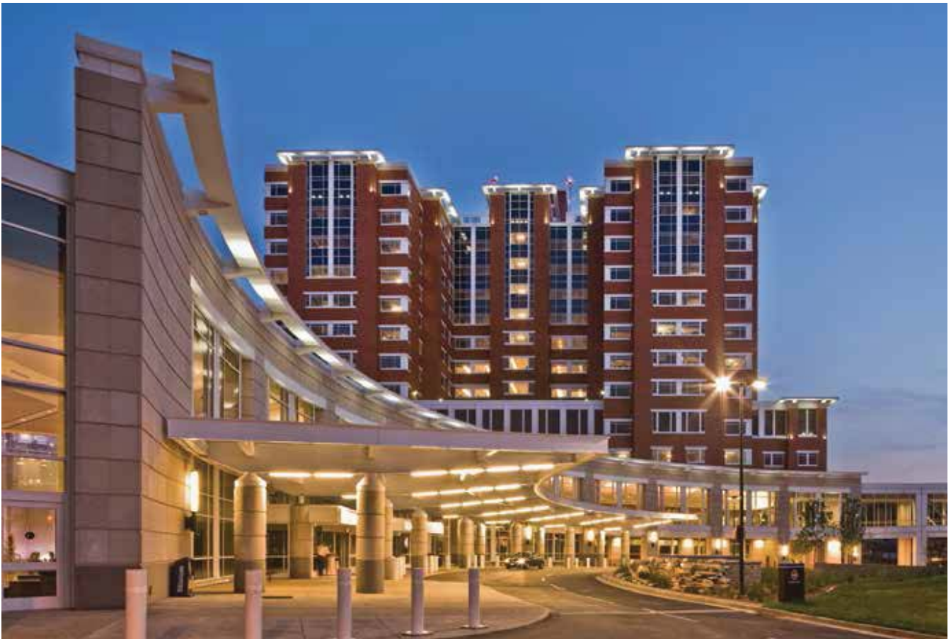
The new 1.2 million square-foot Pavilion A at the Albert B. Chandler Hospital at the University of Kentucky was designed as the new entry point for the complex, connecting to three existing facilities. Precast concrete insulated sandwich panels helped the building meet a number of its goals. Photo Pease Photography, courtesy of GBBN Architects and AECOM.
